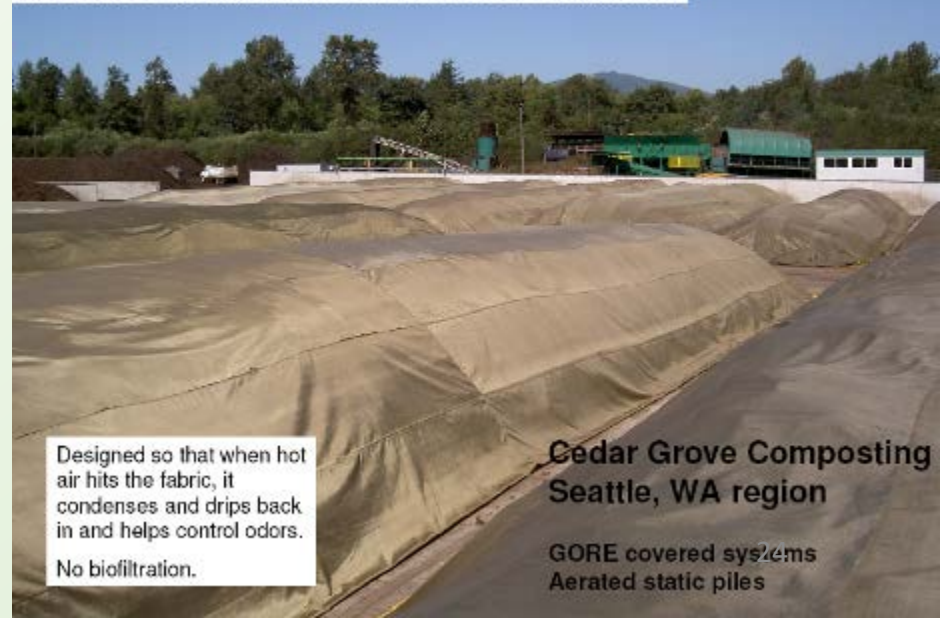
Aeration trenches under the Gore covers. Three phase composting. 2 phases under the covers + 1 curing phase.
